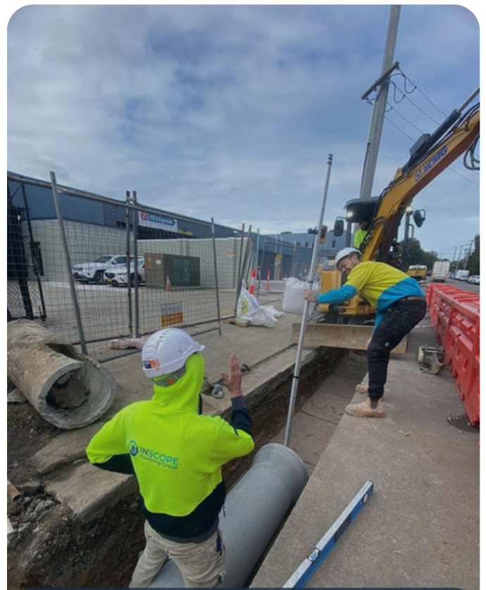
Stormwater pipe installation — Kingsgrove
